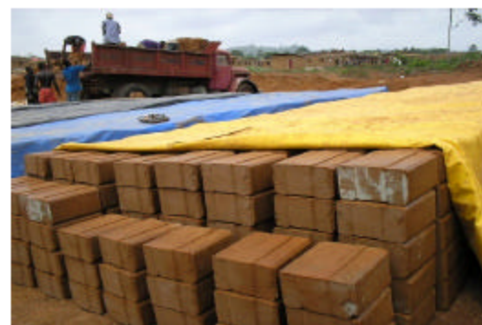
Fig. 3: Stacking and curing of interlocking blocks. Source: Field survey (2007), Obasanjo low-cost housing estate, Ado-Ekiti
