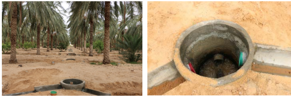
Fig. 3: Water distribution by buried pipeline
